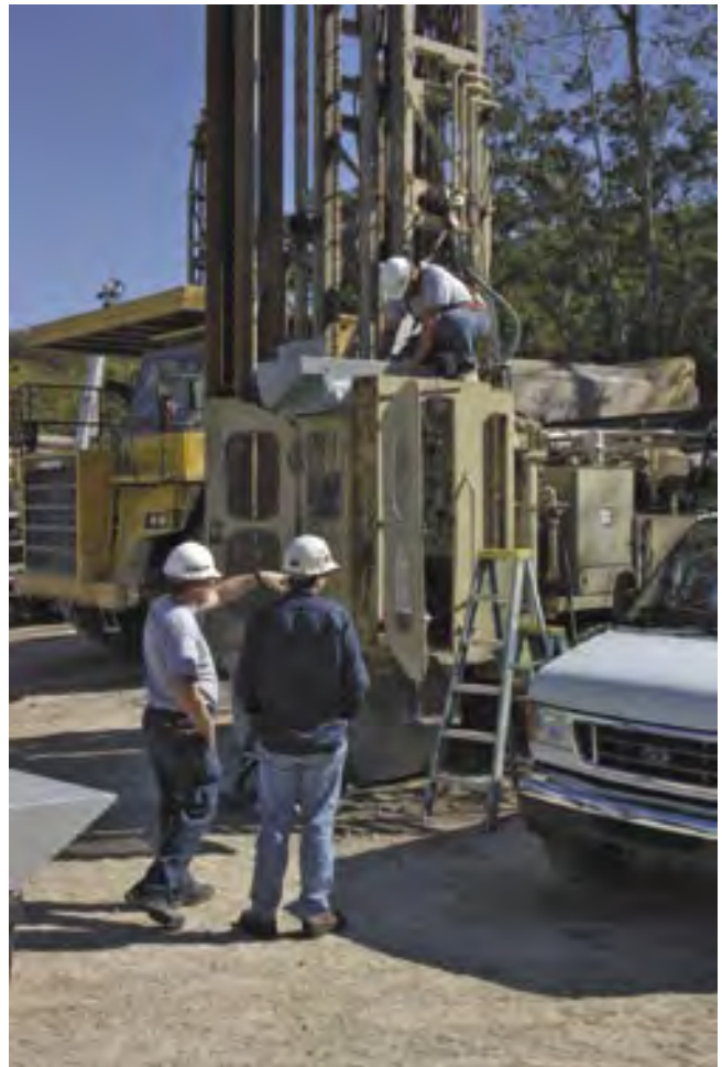
These drill operators are busy installing a new unidirectional filtration and pressurization system.
