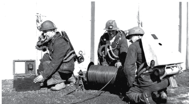
Figure 1, 1940s sound-powered mine rescue communication system
