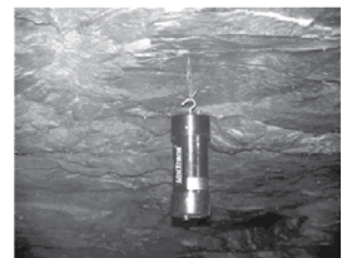
Radio Repeater Underground
