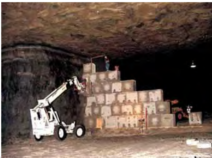
Figure 6: Placing Blocks in Place for Super Stopping.
