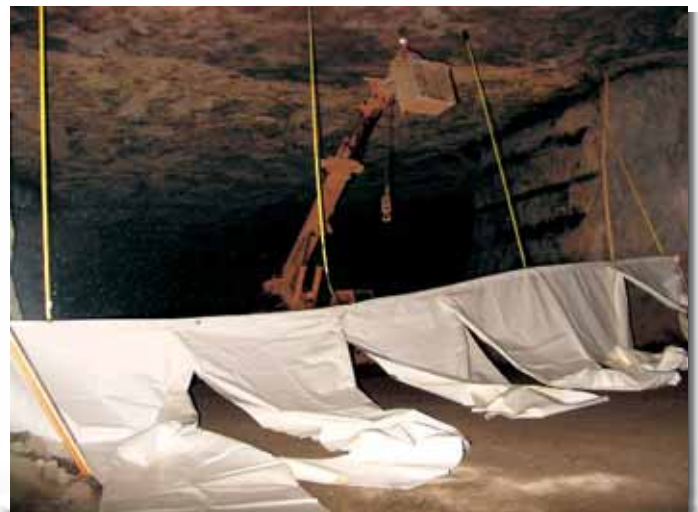
Figure 7: Raising the EZ-Up Stopping.
