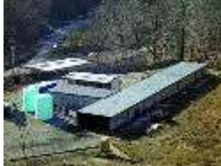
The Fire Suppression Facility (FSF) at Lake Lynn.
