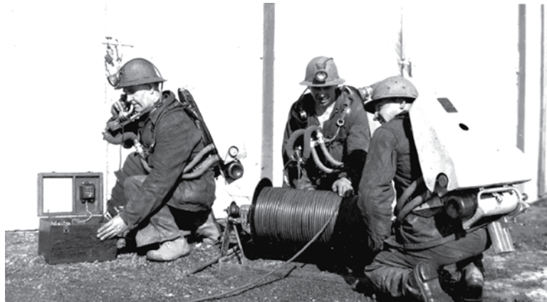
Figure 1, 1940s sound-powered mine rescue communication system
