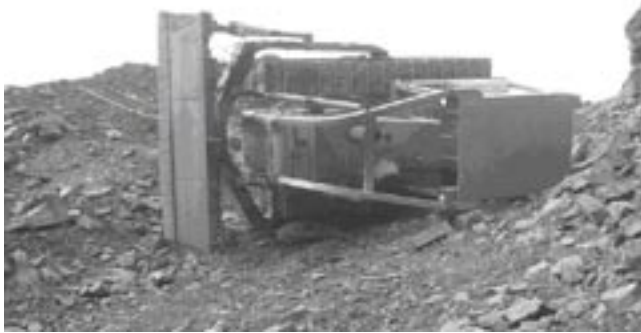
Figure 1. The dozer overturned when the right side track traveled over a partially buried rock
