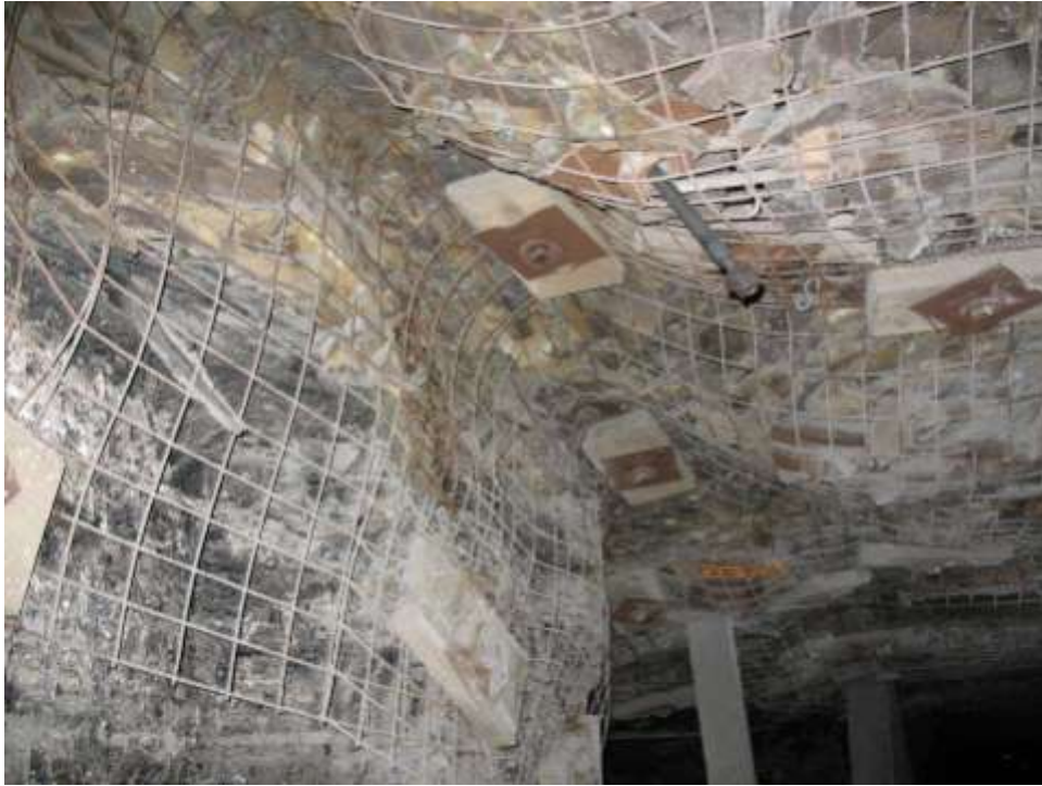
Figure 18: Full screening down the rib protects exposed corners and prevents rock falls.
