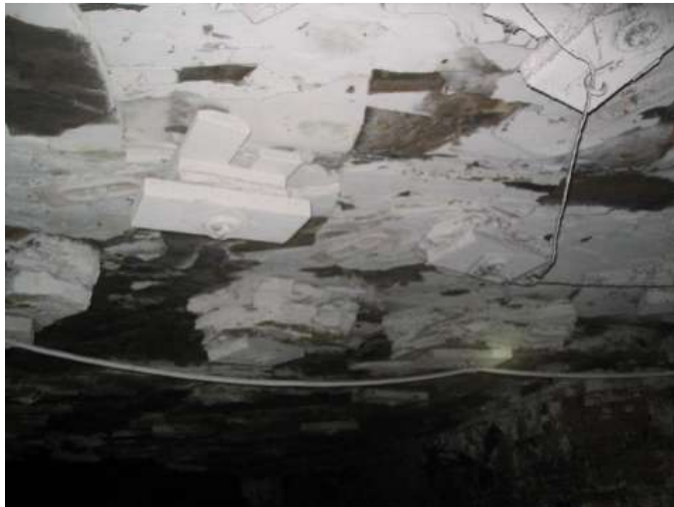
Figure 14: Pinchout of black shale leaves moisture-sensitive gray shale exposed.
