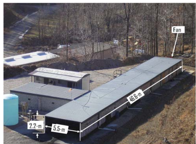
Figure 1. Exterior of Fire Suppression Facility
