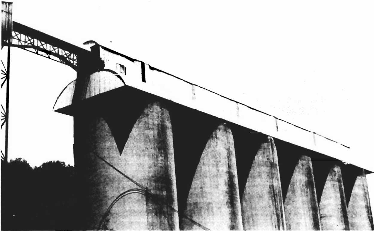
FIGURE 3. - The Nelms No. 2 cluster of open-top silos is covered by a metal roof that allows free movement of air.
