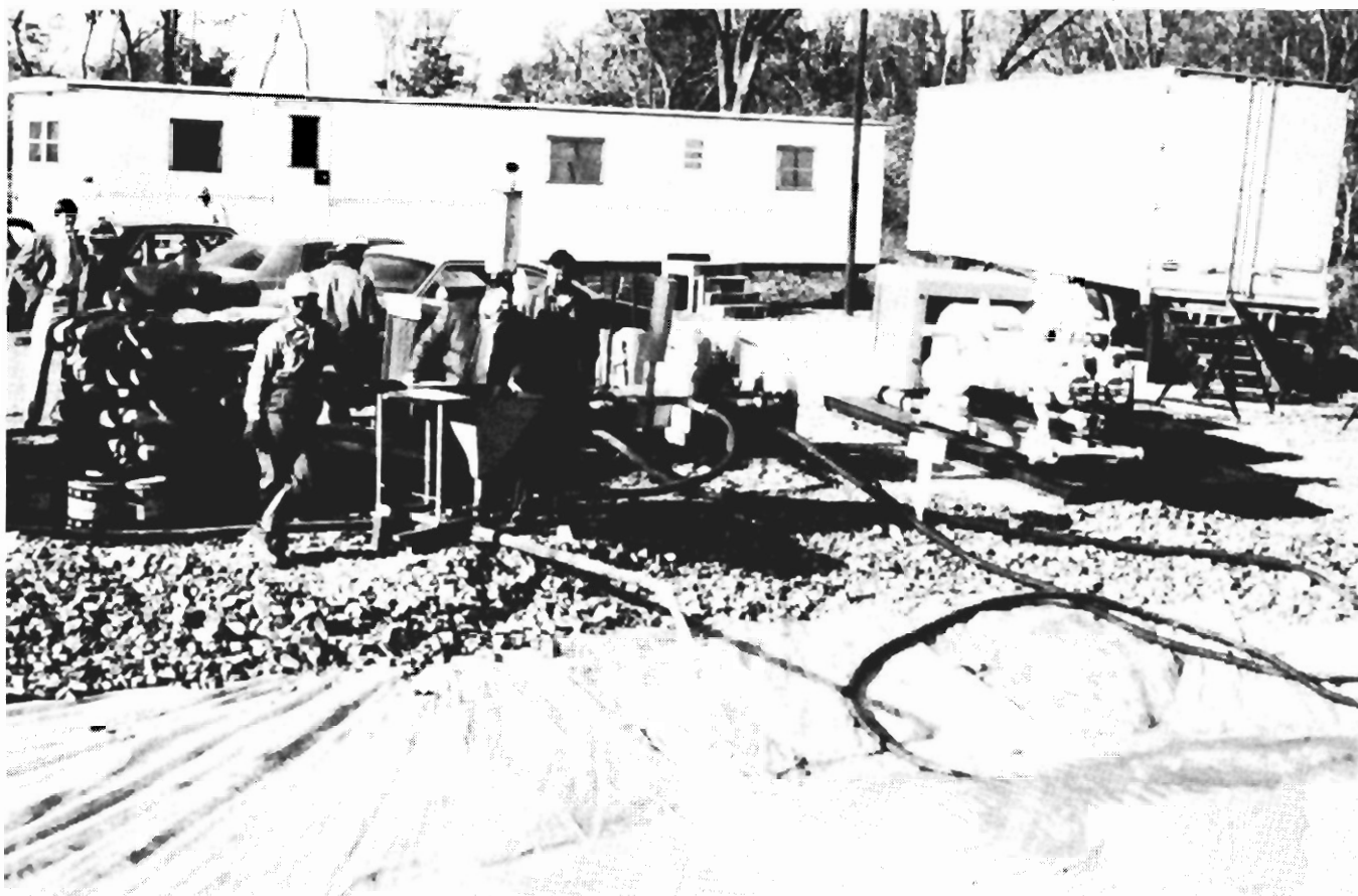
FIGURE 10. - Mixing Dextrid-Polymer mud for pilot hole drilling. Sacks of Dextrid at left, FWI pumps at center, and Gardner-Denver pump at right.
