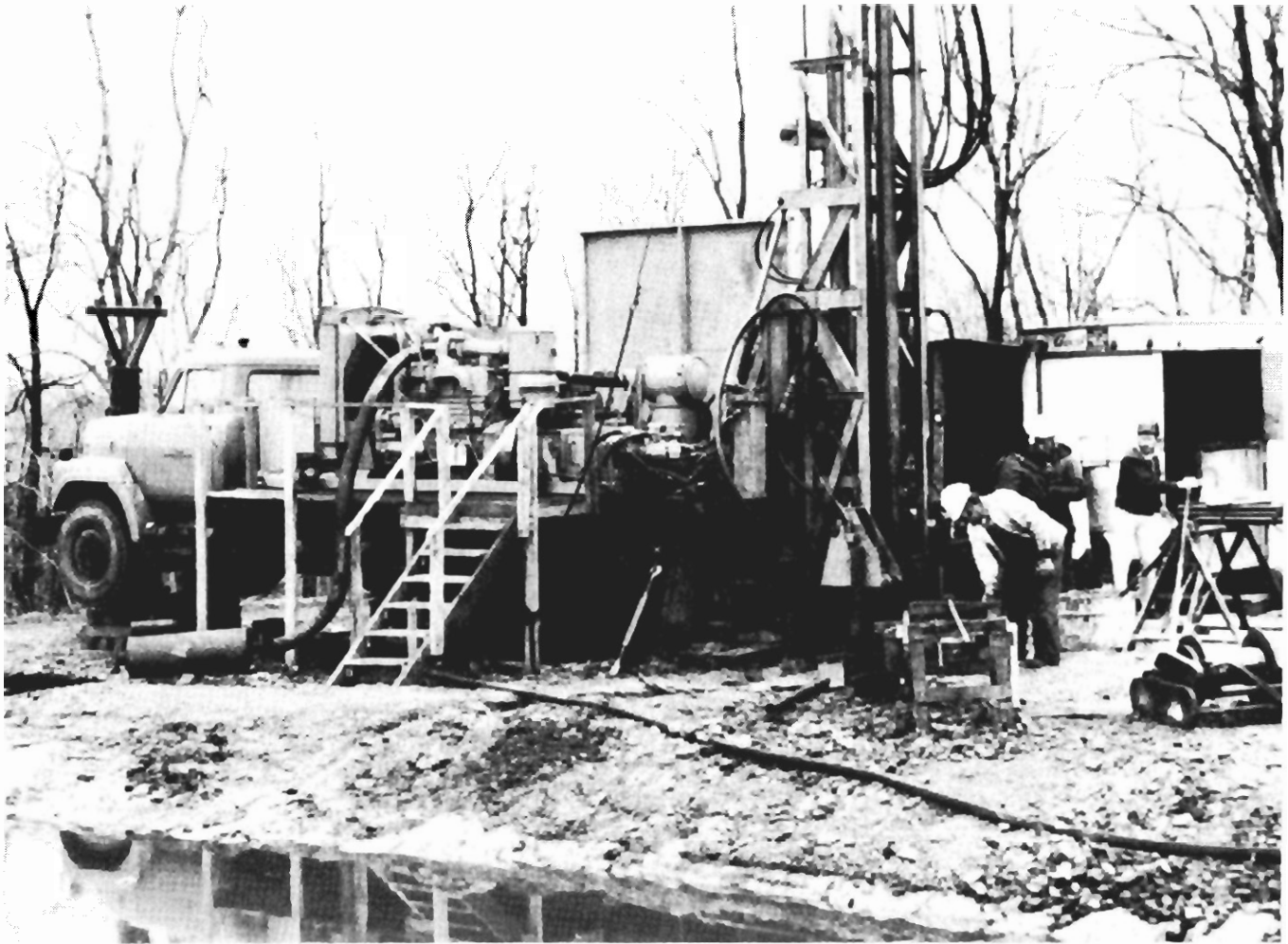
FIGURE 6. - Drilling rig. Note survey tool and wireline hoist in right foreground. Photograph taken during pilot hole drilling operation, November 1978.
