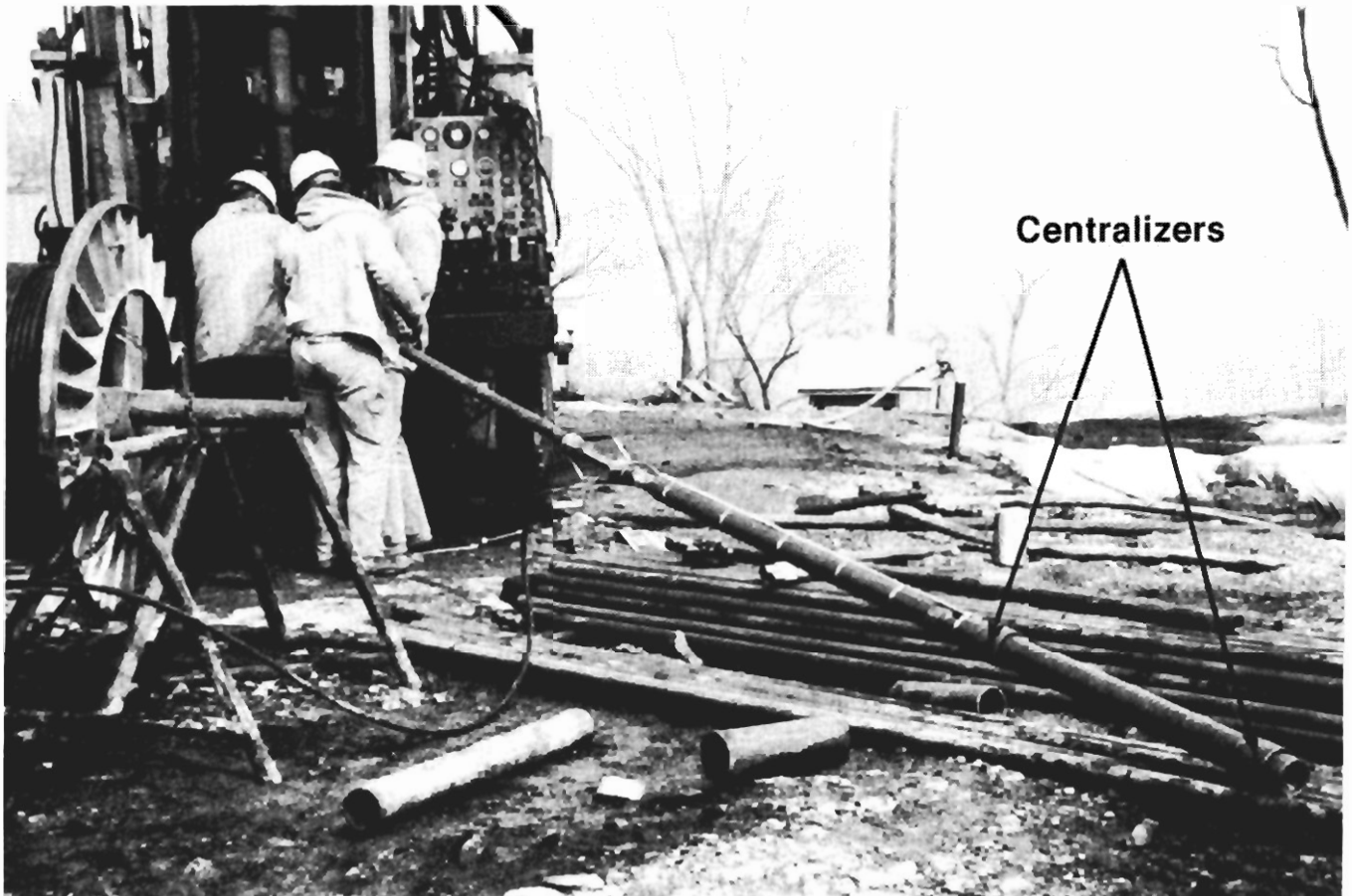
FIGURE 24. - Crew running the submersible pump into EM-19. Note centralizers for motor at right.
