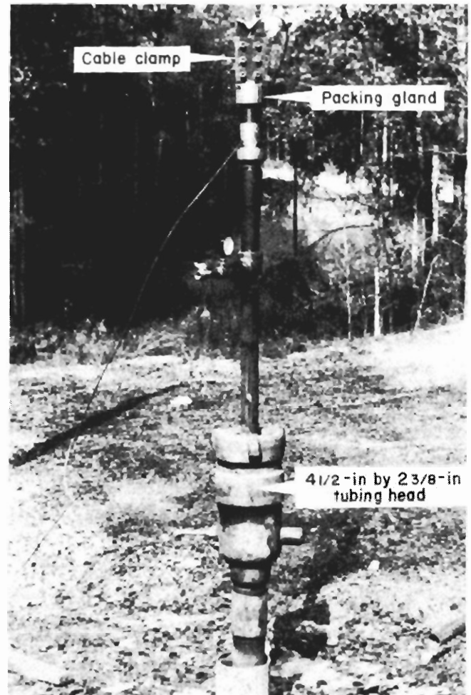
FIGURE 5. - Wellhead assembly.
