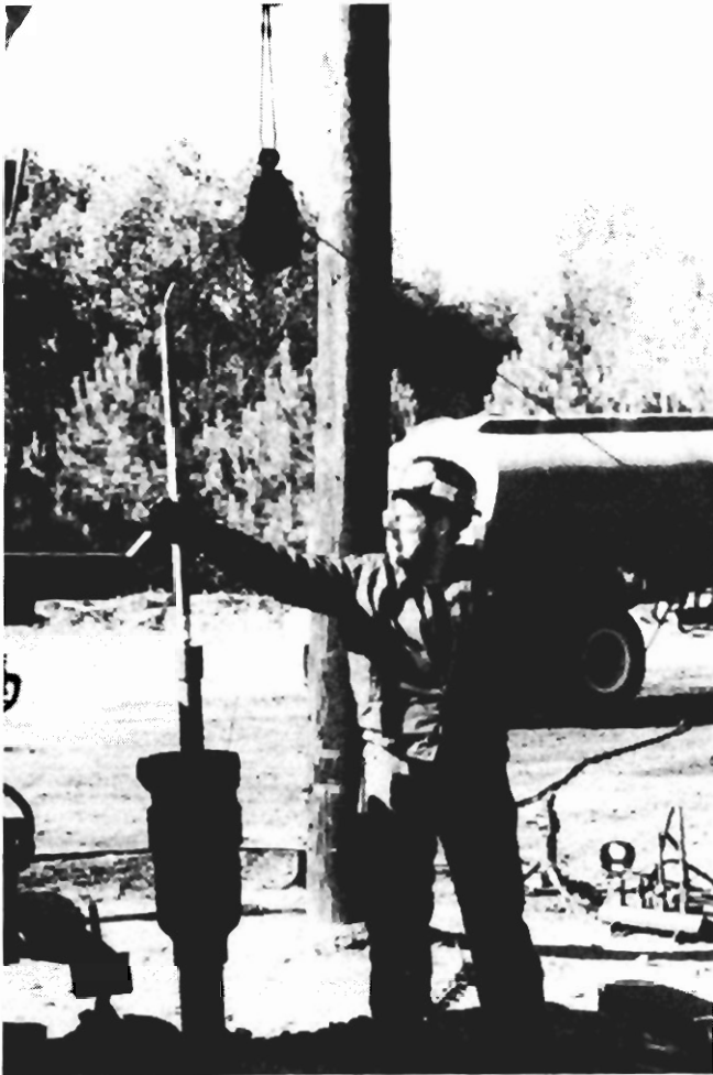
FIGURE 4. - Sentry unit being installed in monitor hole M3.
