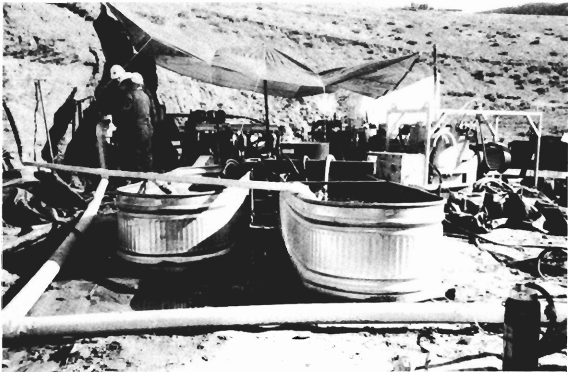
FIGURE 3.—Navajo Dam demonstration borehole drill site.
