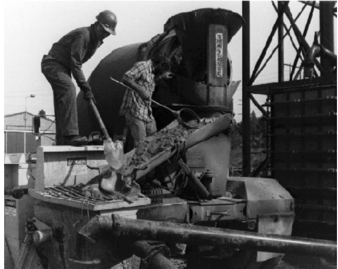
Transferring total tailings paste backfill from ready-mix truck to pump hopper.
