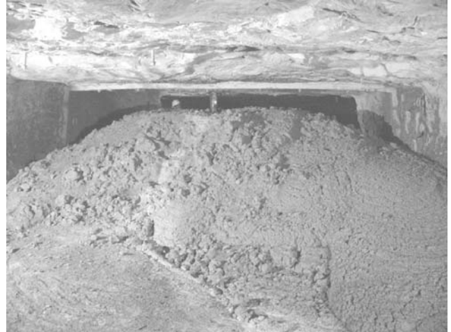
Figure 8. View of bulk fill placement for seal No. 2.
