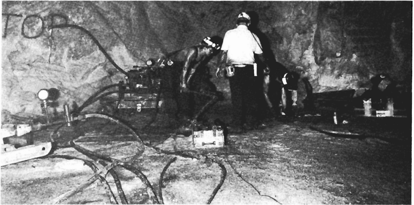
FIGURE 24. - Equipment assembly for exploratory drilling in study area.
