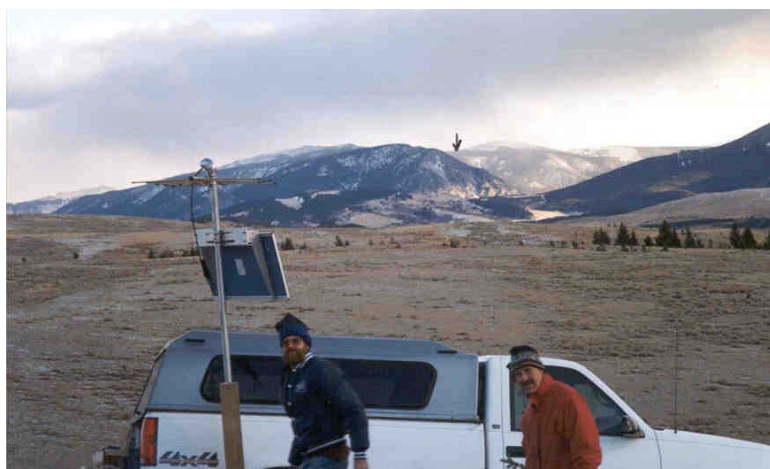
Figure 2. Mission Creek repeater station
