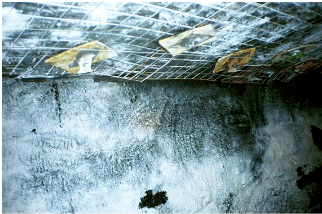
Figure 2. Roof screen achieving up to 94% roof coverage.
