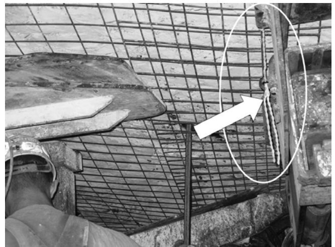
Figure 5. Roof screen held in position on ATRS with twisted 12-gauge wire.
