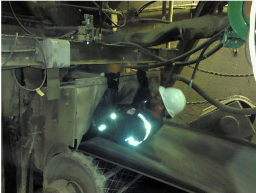
Fig. 1. Entering mixer drum to perform maintenance
