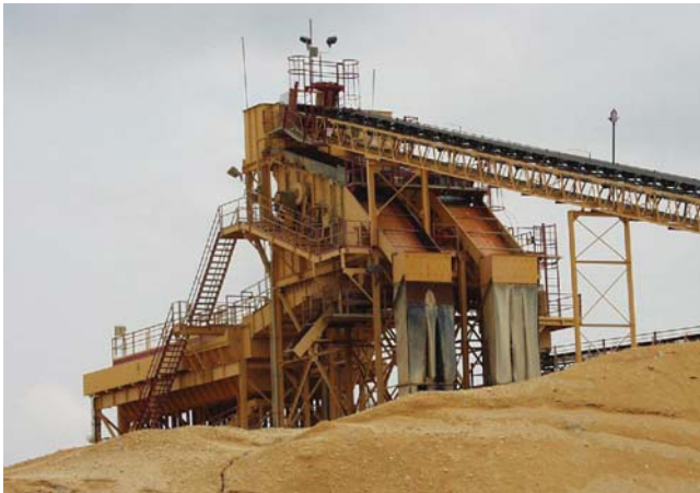
Diester 1.8- x 6.1-m (6- x 20-ft) shaker screens.
