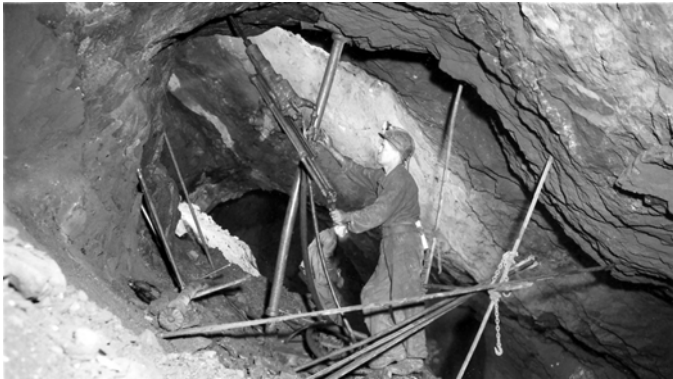
Figure 1. Angle drilling in an open stope.
