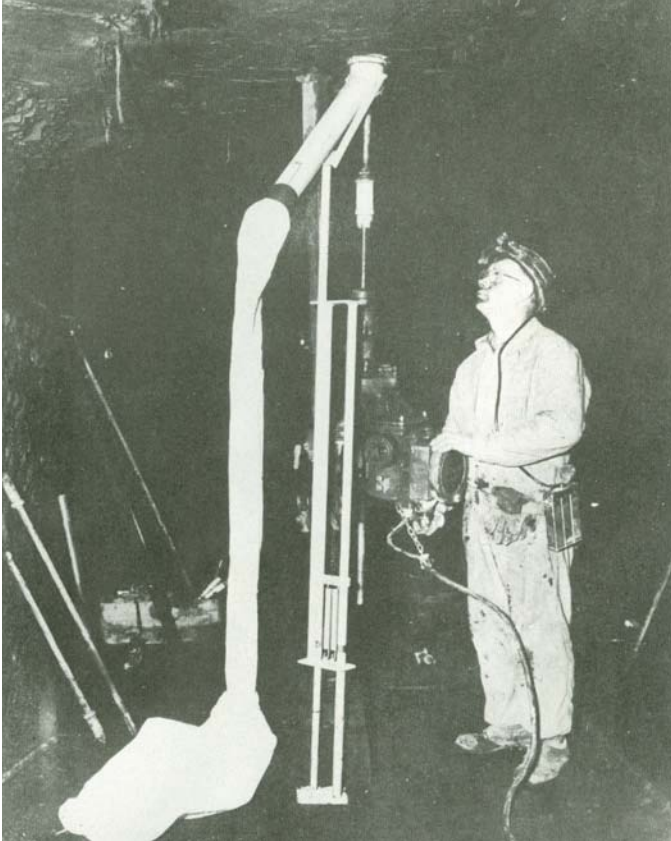
Figure 5. Testing a Browning dust collector.
