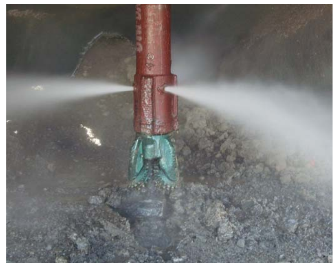
Figure 9. Water separator sub with rotary bit.
