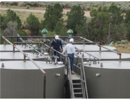
Workers inspect oil production tanks. Photo from NIOSH
