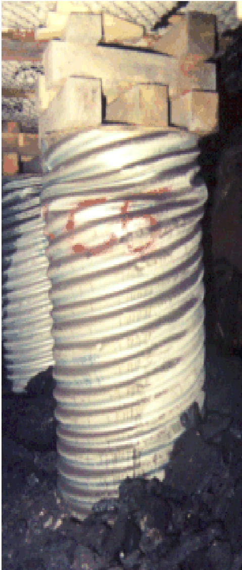
Figure 2. Confined Core Crib (3C) support was the first viable alternative to wood cribbing in western longwall tailgates.
