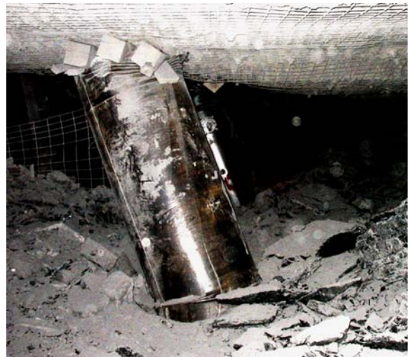
Figure 6. The Can is the most stable support presently available. It can accommodate large roof-to-floor convergence as well as large lateral displacements.
