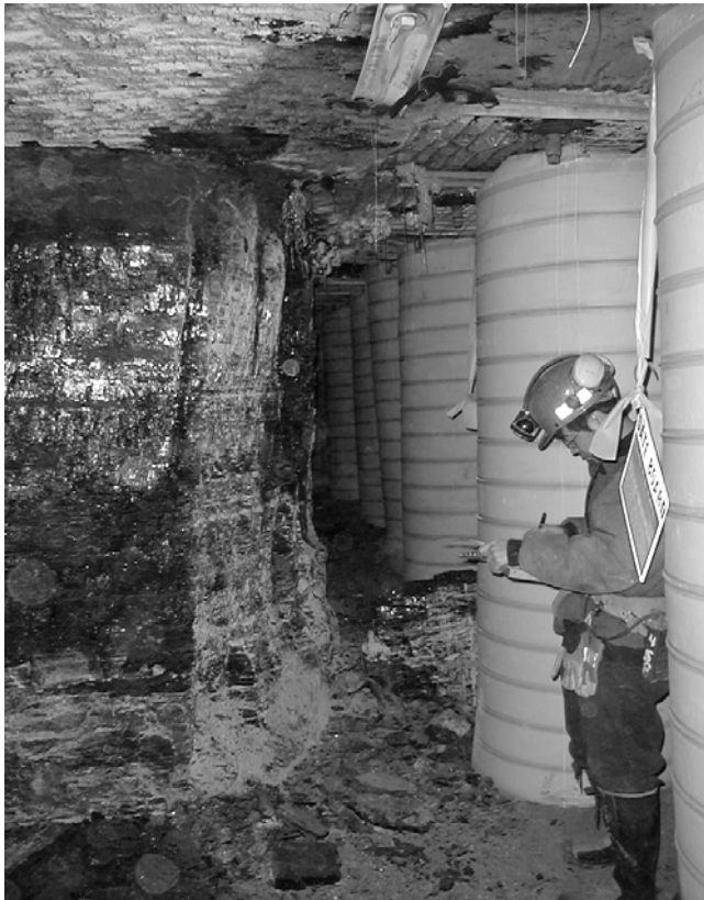
Figure 11. Visual observations were made and recorded routinely throughout the investigation.
