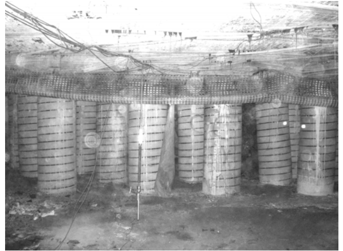
Figure 7. Looking inby the C chute. The Serata closure meter is installed and recording roof-to-floor closure.
