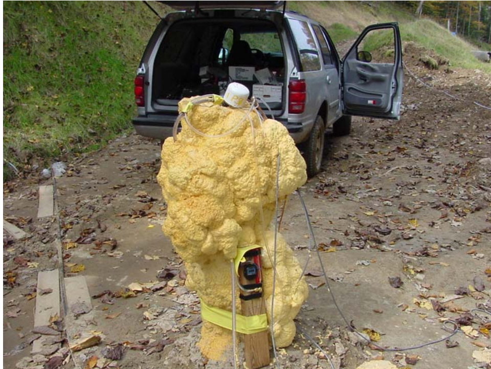
Figure 5. A pressure sensor mounted on top of borehole. Polyurethane foam was used to seal the borehole.
