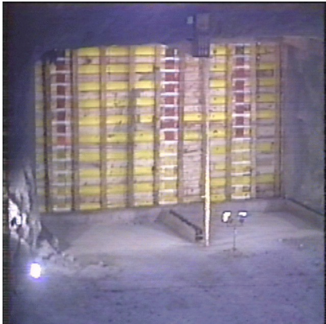
Figure 11. Mine seal just prior to explosion test.
