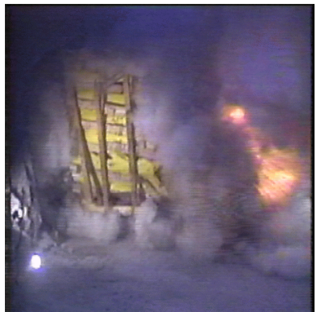
Figure 14. Complete failure of seal.
