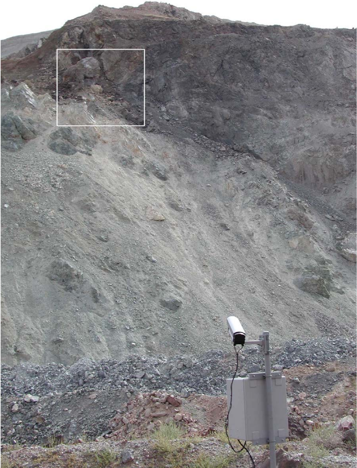
Figure 4.—Highwall at the Yellowstone Mine showing area monitored by video camera (white box).
