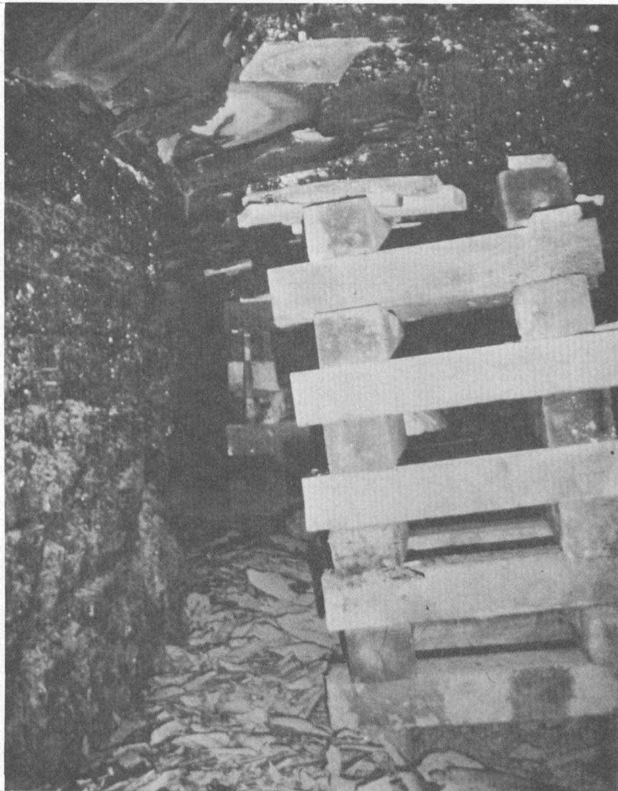
FIGURE 23. - "Cutter" occurring parallel to the rib.
