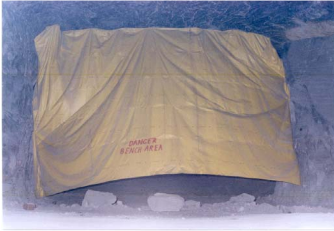
Figure 11. Leakage through brattice stopping
