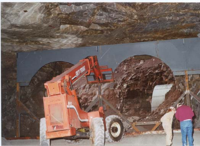
Figure 7. Installation of prefabricated fan bulkhead
