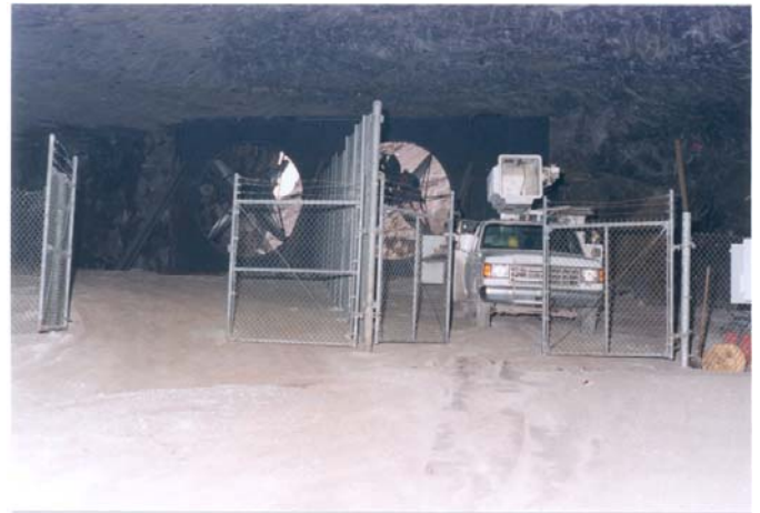
Figure 8. Fan installation with perimeter guarding during maintenance.
