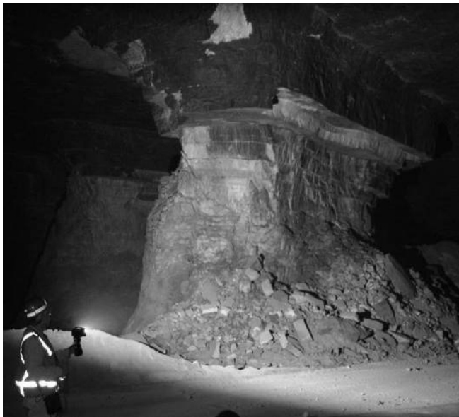
Figure 5. Pillar instability observed in Mine B, showing the influence of weak bedding layers (Case 7 in table 5).
