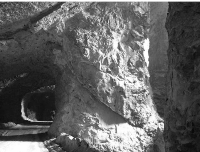
Figure 7. Pillar instability caused by a continuous geological structure cutting through the pillar at Mine D. Thread-bar bolts that were installed right through the pillar are visible (Case 4 in table 5).
