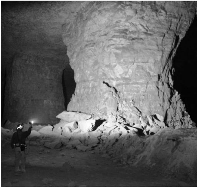
Figure 6. An unstable pillar at the edge of benching operations at Mine C, showing the effect of brittle failure and spalling resulting in an hourglass shape (Case 5 in table 5).
