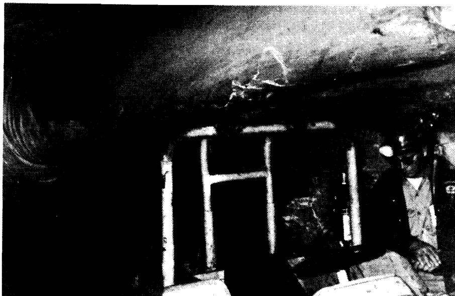
Figure 4-31. Underground Mine Canopy Clearance Problems
