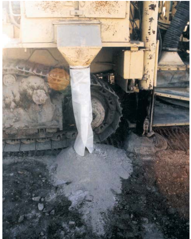
Dust collector dump shroud after installation.
