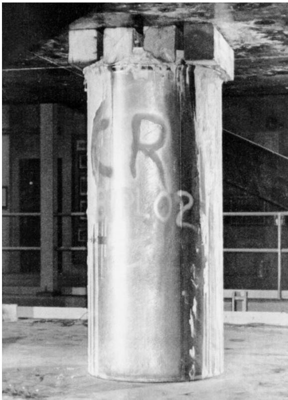
Figure 5.—Can crib used to replace wood crib in underground coal mines.
