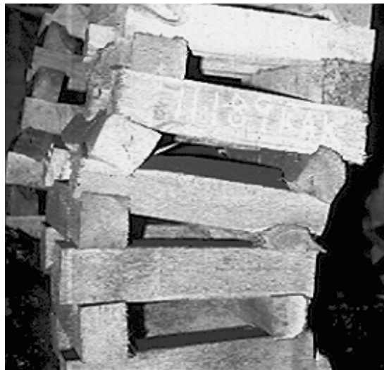
Figure 1. Instability in 4-point wood crib caused by single soft timber
