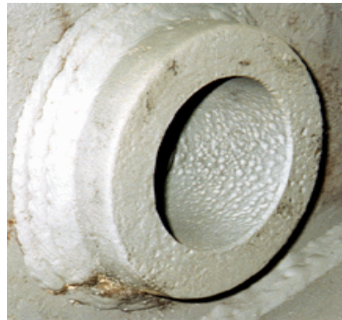
Figure 15. Corrosion of a lemniscate link bore can significantly increase the stress from link loading and increase the probability of failure
