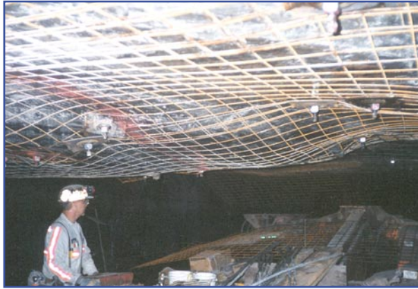
Roof screen can cover a large area of the mine roof.
