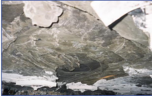
Loose rocks can fall from between roof bolts and injure miners.
