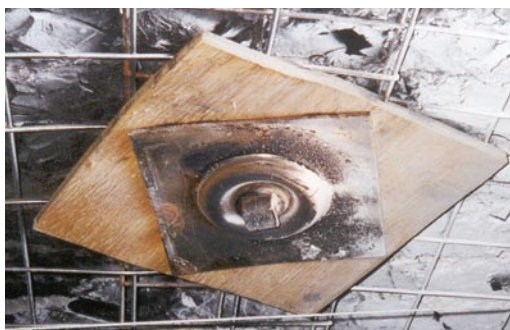
Plywood installed between roof bolt plate and roof screen.
