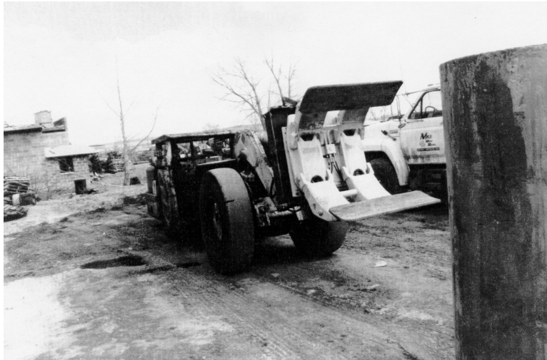
Figure 8.— Attachment used to pick up and maneuver can cribs.
