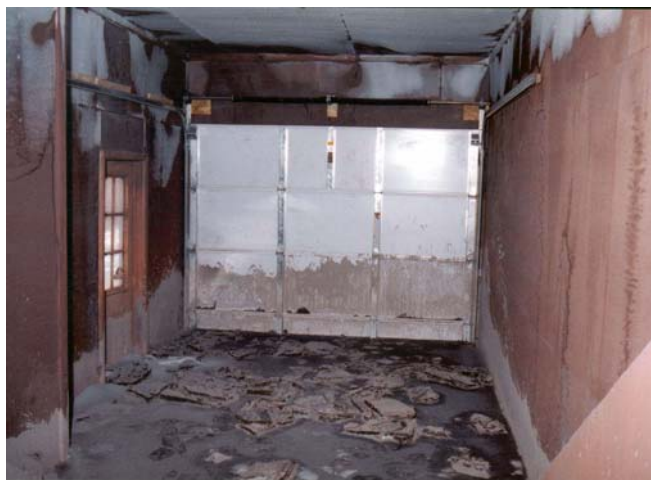
Figure 3a. Seal replaced at eastern end of reclaim tunnel to access outside
