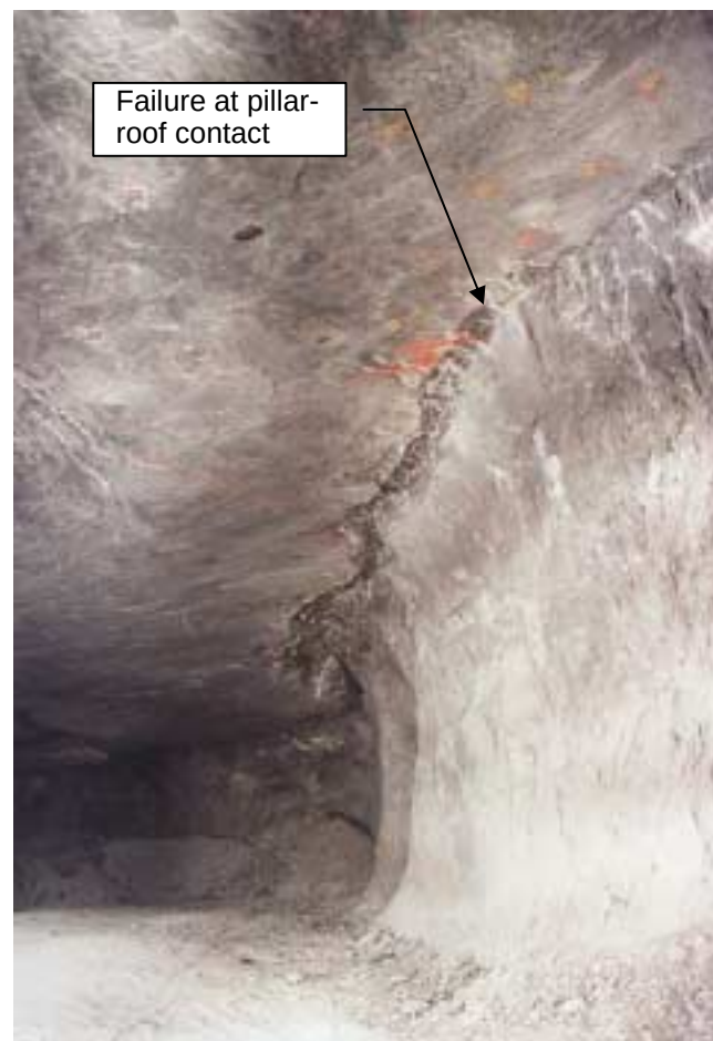
Figure 1. Photograph showing failure at pillar-roof contact after loose rock has been removed and roof has been re-supported.
