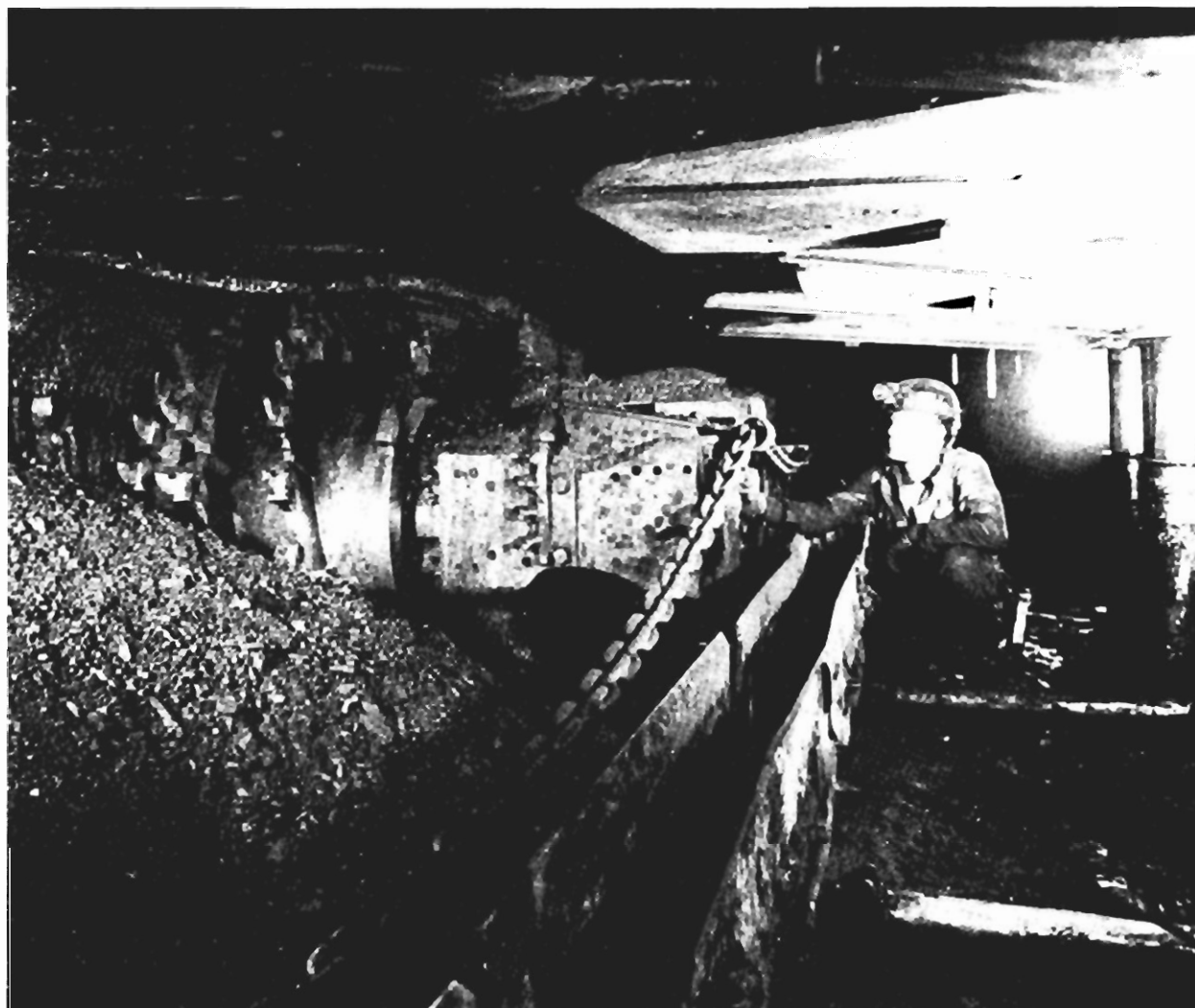
FIGURE 18. - Illustration of longwall working environment.
