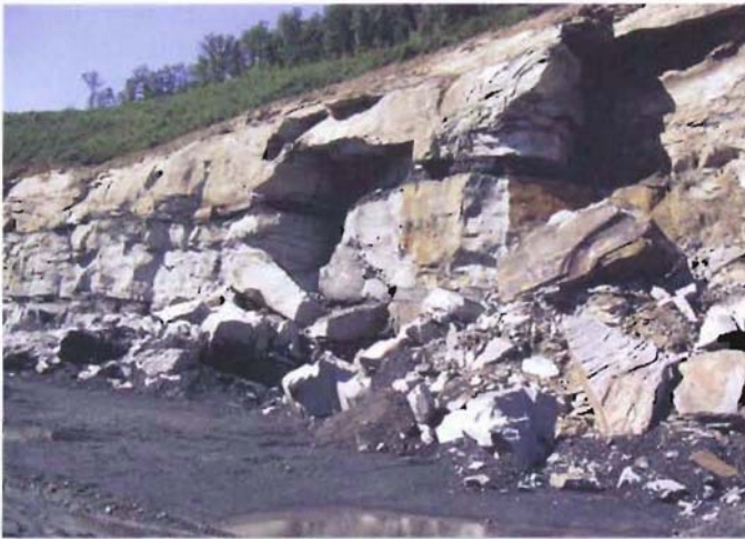
Figure 9—Highwall collapse site.
