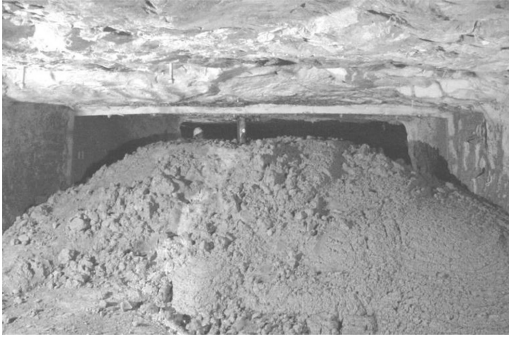
Figure 5. View of bulk fill placement for mine seal.
