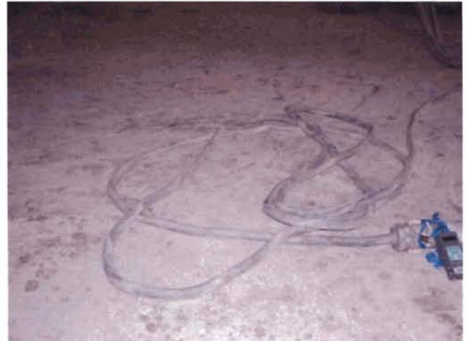
Figure 3a. Shredder cable haphazardly over-lapped.
