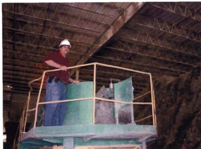
Figure 4a. Shredder tub with door installed.
