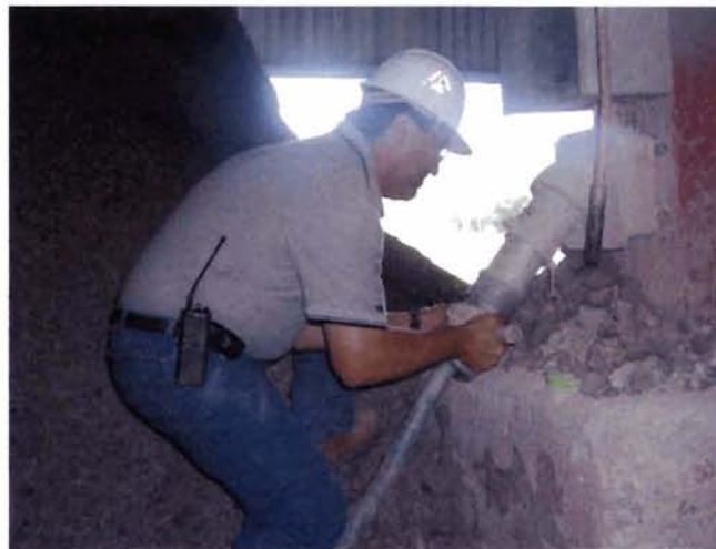
Figure 1. Mine worker demonstrates power connection.
