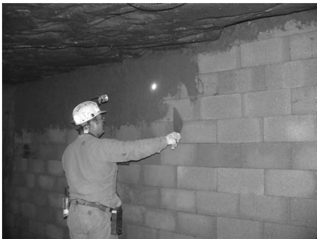
Figure 2. Miner applying sealant to concrete block stopping
