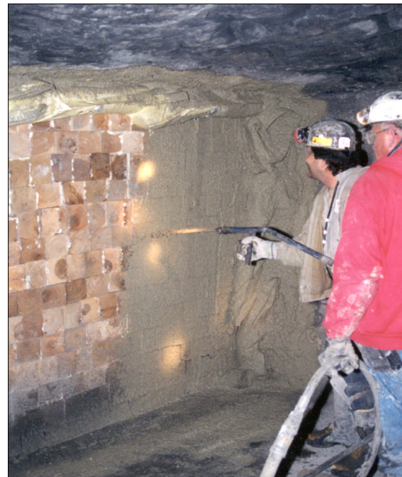
Figure 4- Coating wood seal with Strata sealant
