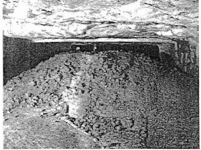
Figure 9 — View of bulk fill placement for seal No. 2.
