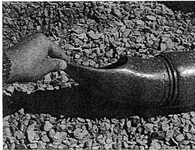
Figure 6 — Elbow for bulk fill placement.
