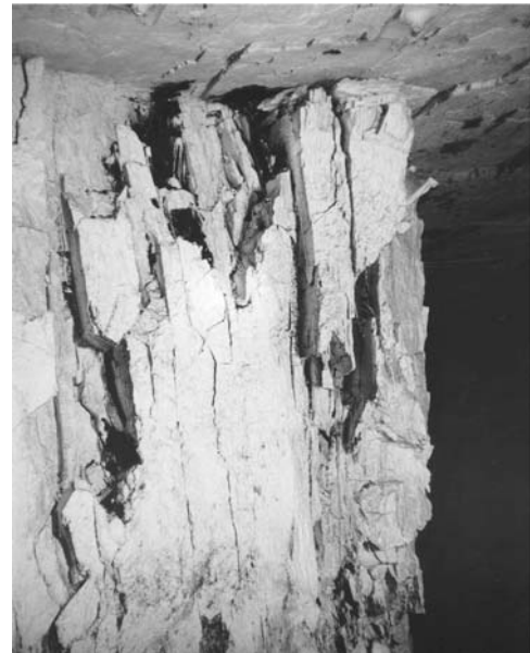
Figure 1. Vertical coal pillar slabs associated with face cleat.
