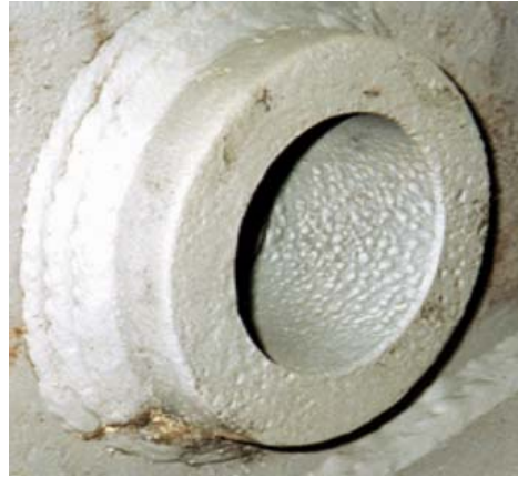
Figure 7 Corrosion of a lemniscate link clevis
