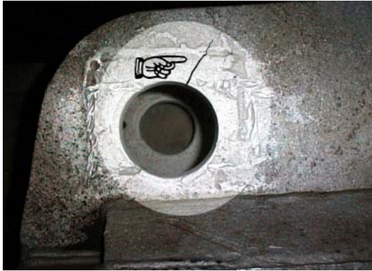
Figure 10. Failure in base lemniscate link clevis
