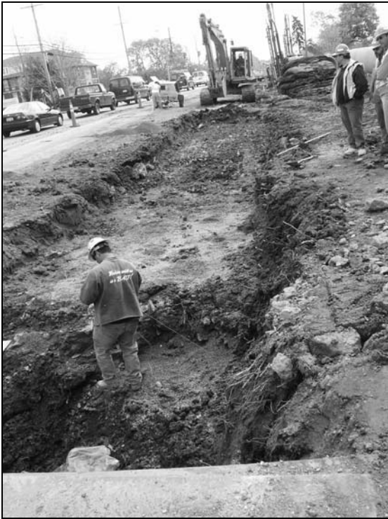
Figure 5 - Overburden is removed from the rock.
