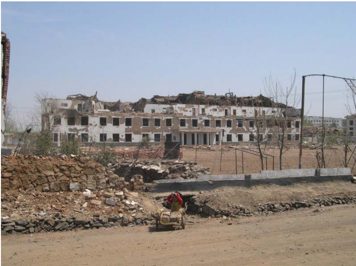
Figure 3. Ryongchon Primary School was severely damaged by the train explosion.
