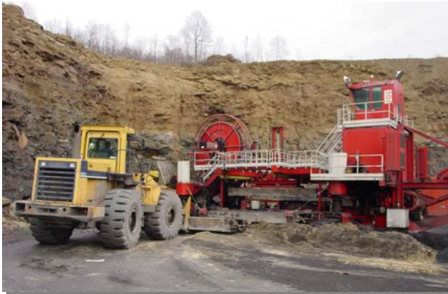
Photograph 1. "Push beam" being loaded into a SHM.
