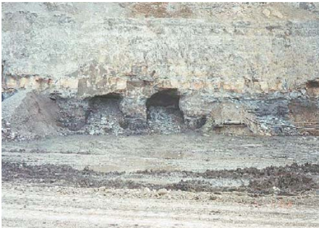
Photograph 4. Roof Falls and Web Collapse
